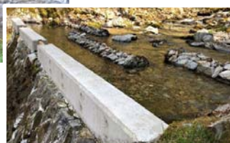
(取水堰改修後)
